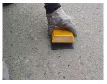
As with all sealent materials, contacting surfaces must be completely clean, dry and free of foreign and loose materials. When used for repairing cuts in existing pavements, openings should be squarely and
